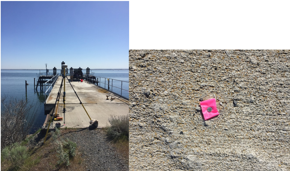
Figure 2. Temporary control point (TCP) establishment.
