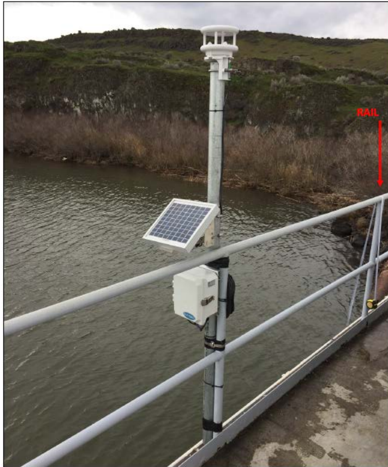
Figure 3. Water level data collection platform with wind sensor.
